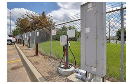
AUI installed four Leviton Electric Vehicle (EV) chargers at its Head Office in the fall of 2021. These chargers are level 2, meaning they can fill most EVs within five hours from empty.
